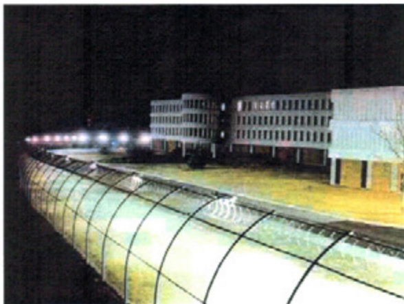
Figure 22. Instant-on, reflectorized fluorescent prison lighting appears as a “wall of light” to inmates. Patrol personnel and vehicles cannot be detected during patrol. (Photo courtesy of Magnaray)
