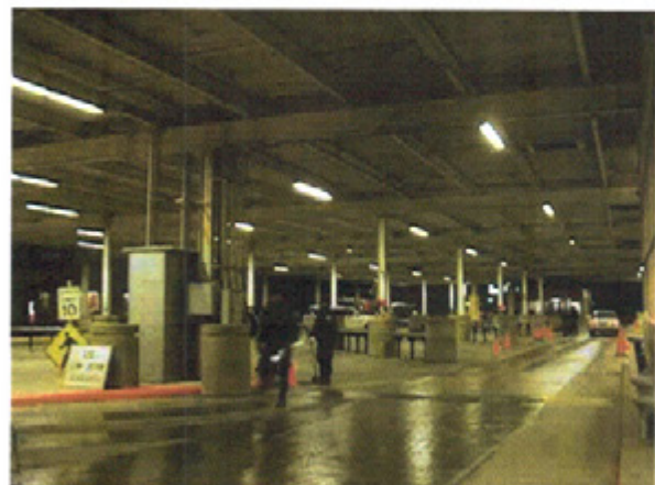
Figure 7. Uniform lighting in areas where pedestrians interact with moving vehicles may provide better visibility. (Provided courtesy of Magnaray® International Division)
