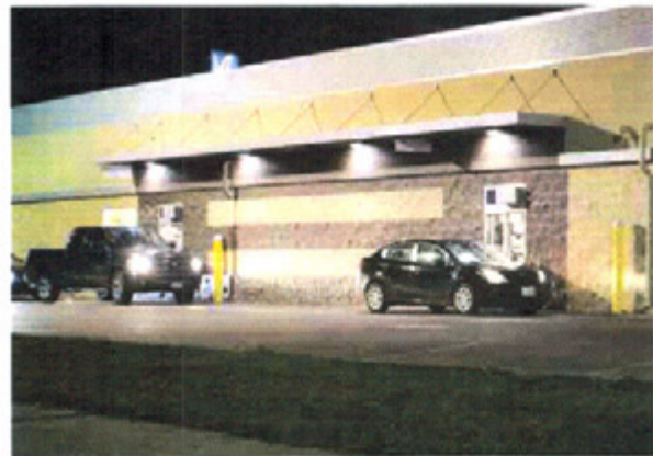
Figure 26. In this example, recessed luminaires define the building with a soft wash of light and highlight the drive-up window, allowing window-service personnel to clearly see the arriving customers. Light-colored surfaces reflect light onto the driveway for easy wayfinding.
