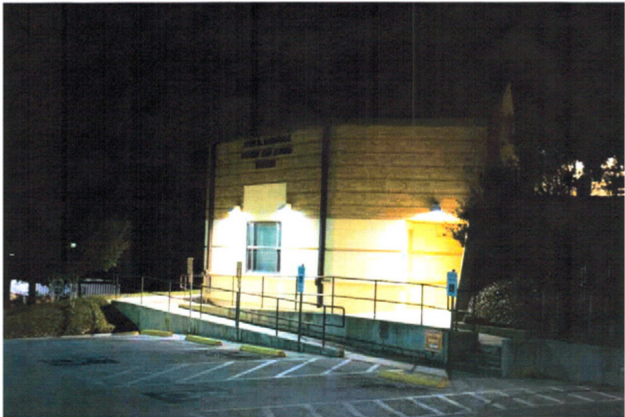
Figure 33. Lighting for vehicular and pedestrian traffic facilitates surveillance when security issues are a high priority on campus. Compare and contrast with the dark side of the building, which was not considered in the lighting design. (Photo courtesy of OSS – Law Enforcement Advisors ® )
