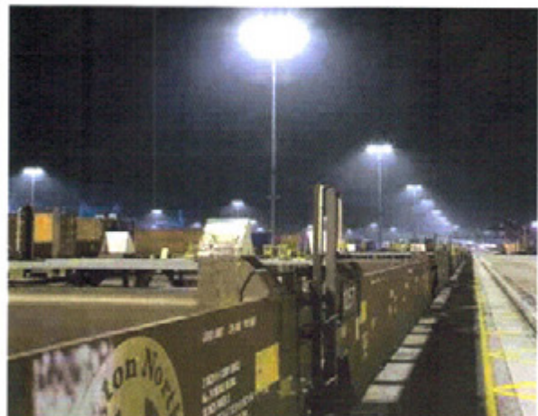
Figure 17. Area lighting for storage yards, industrial parks, and truck and rail terminals, often supported with floodlighting or luminaires mounted on poles. (Photo courtesy of Acuity Brands)
