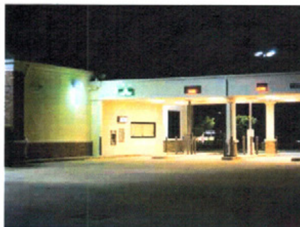
Figure 20. Recessed luminaires in the roof overhang provide uniform lighting on the walkway and vertical illuminance for customer transactions at the machine. (Photo courtesy of OSS – Law Enforcement Advisors ® )
