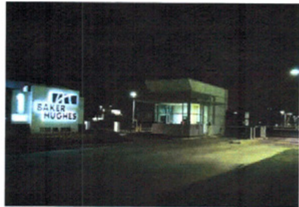
Figure 13. Driveway approach and canopy at the guardhouse provide uniform light for checking vehicles. (Photo courtesy of OSS – Law Enforcement Advisors ® )
