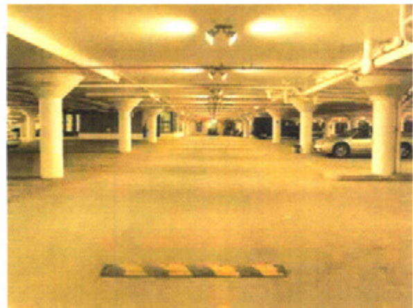
Figure 23. Multiple structural elements coupled with a low ceiling can make it difficult to achieve uniformity, especially between parked cars. In this example, the designer was successful. (Photo courtesy of Larry Leetzow)
