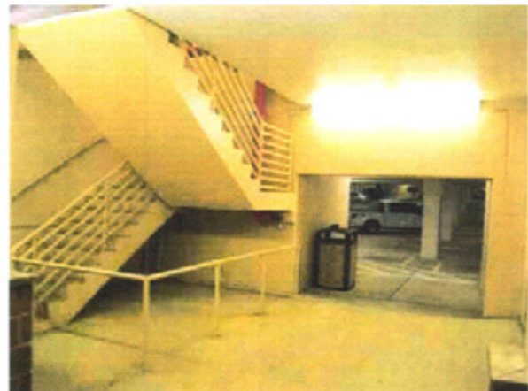
Figure 24. This well-lighted stairwell will create a greater sense of safety and security for those who use it. (Photo courtesy of OSS – Law Enforcement Advisors®)
