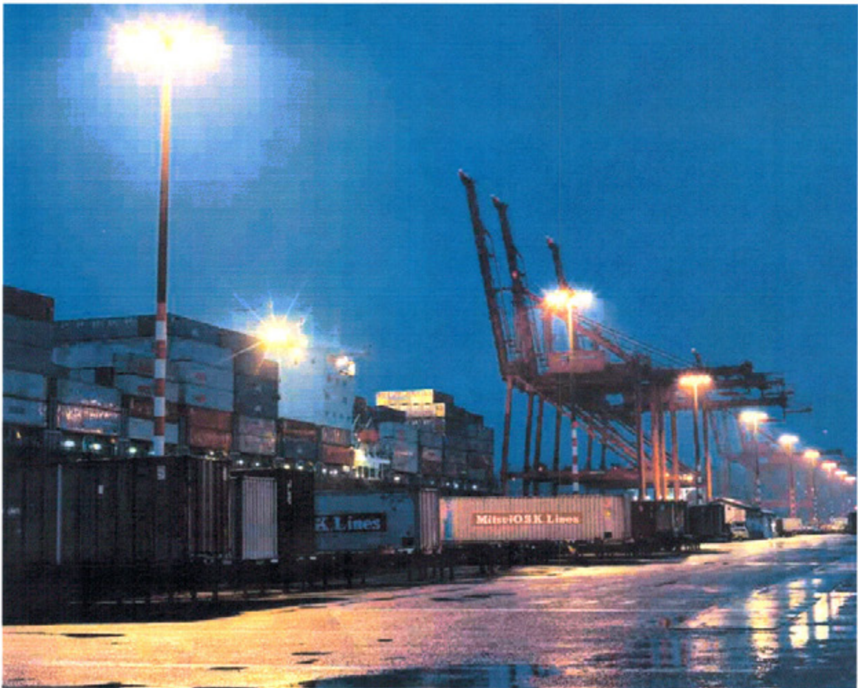
Figure 8. Uniformly spaced poles and luminaires provide lighting at each crane assembly area in this cargo terminal. (Photo courtesy of Holophane)
