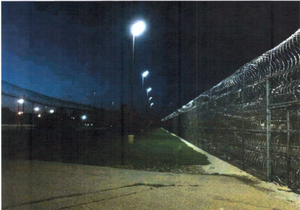
Figure 15. If a view through the barrier is desirable, a set of pole-mounted fixtures set back inside the secured perimeter is effective. (Photo provided courtesy of Magnaray® International Division)
