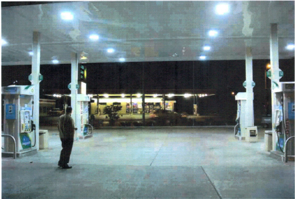
Figure 27. Transition between pump island and service building is facilitated when uniformity ratios do not exceed 4:1. (Photo courtesy of Don Monahan)
