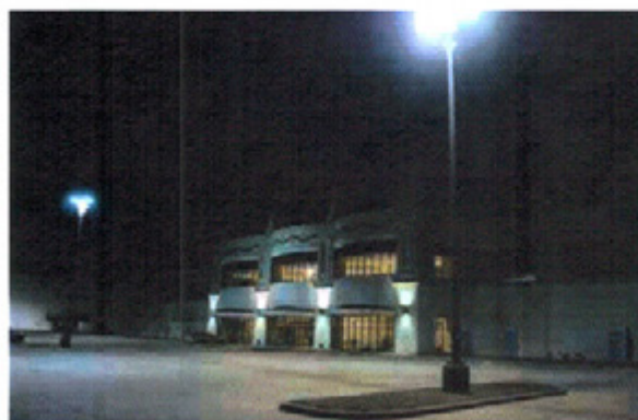
Figure 21. Well-shielded luminaires in an employee parking lot provide uniform illumination for workers leaving after normal business hours and excellent surveillance opportunities for observers from an upper floor in the building. (Photo courtesy of OSS – Law Enforcement Advisors®)
